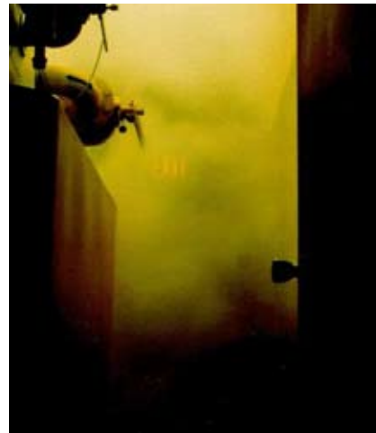
EXIT Sign obscured by smoke
