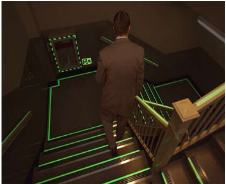
Photoluminescent safety signs and egress systems available from Safety Step Egress glow clearly in complete darkness and illuminate a safe evacuation route when the way out is poorly lit or obscured.
