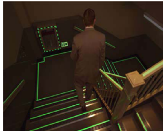
Complete Egress system
